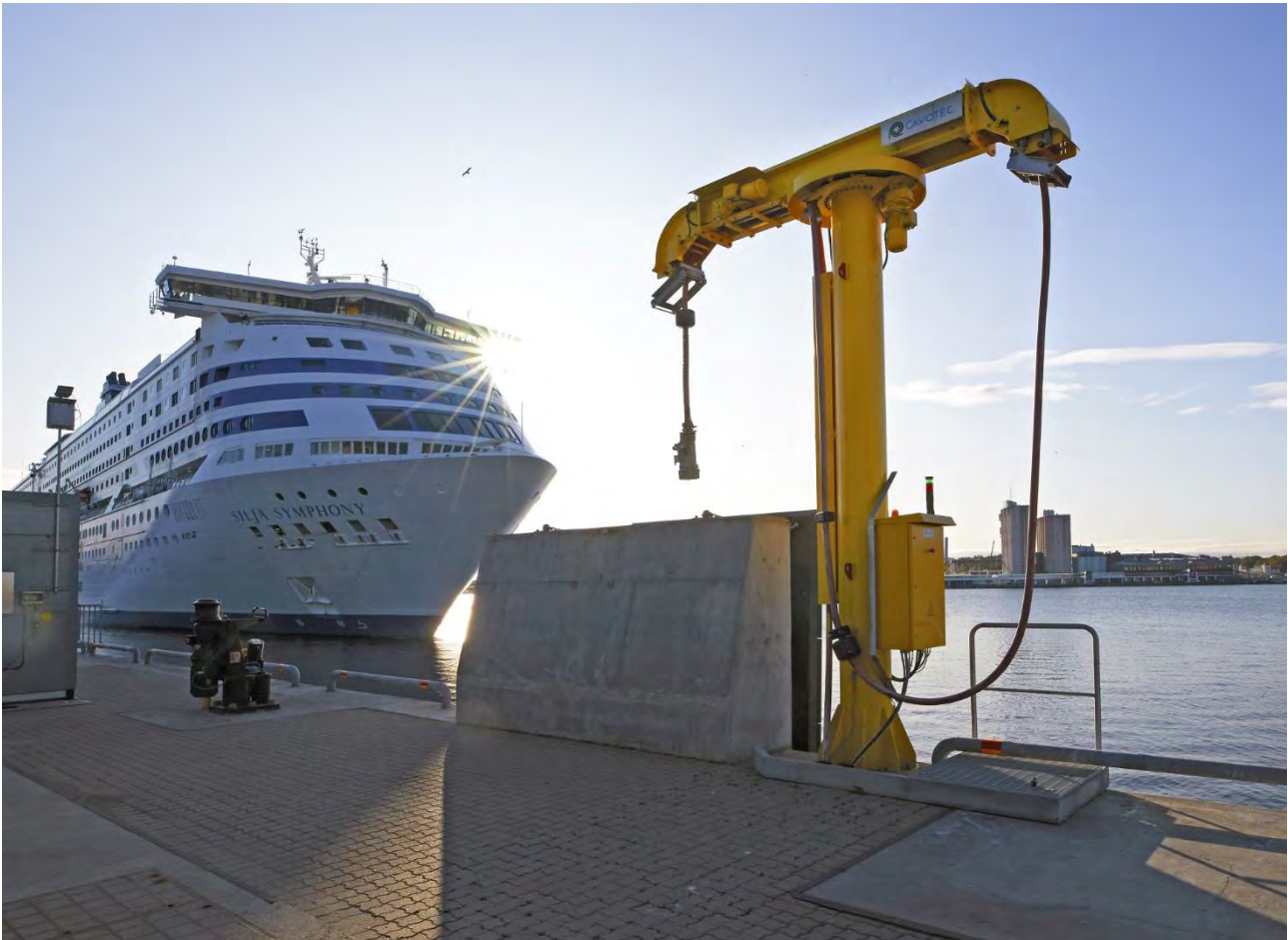
Figure 3 - Port of Stockholm: OPS facilities (source: baltictransportjournal.com)
